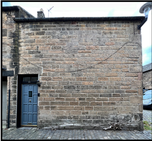
Fig 2 - Front door view of 20 Randolph Lane
